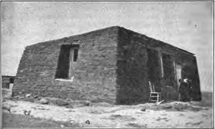
FIG. 4.—Sod house of the new settler on the treeless prairie of North Dakota, built of the resources at hand. Commerce has made the minimum contribution to it. No wooden house is so warm.
